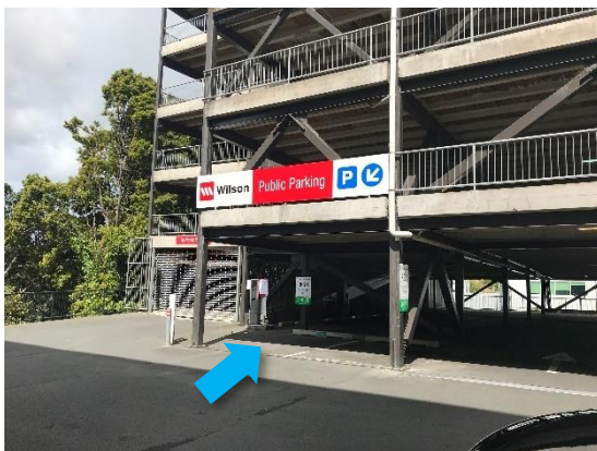
Entrance to parking building
